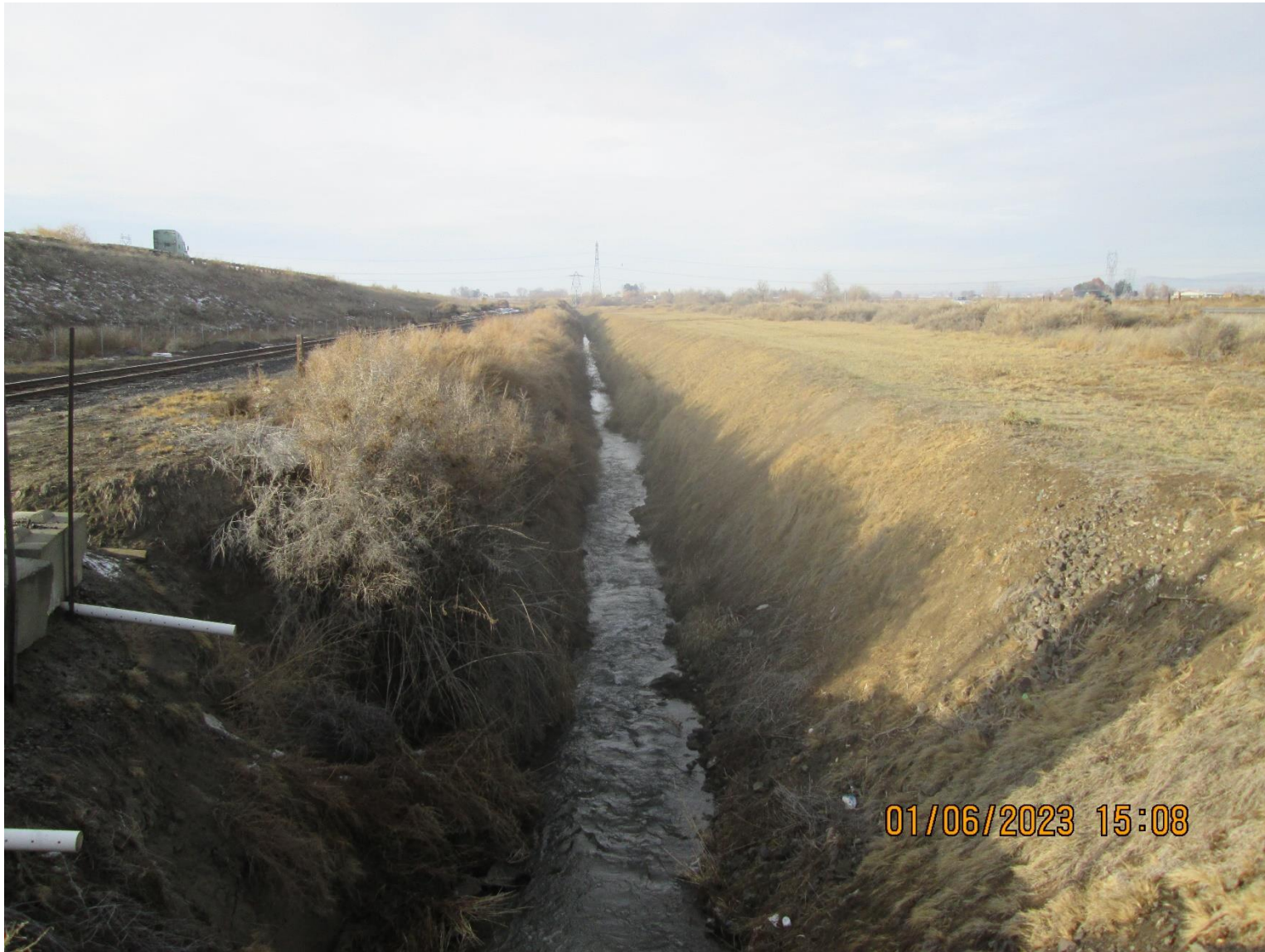
Granger Drain where Gap Road crosses the drain – Looking east
