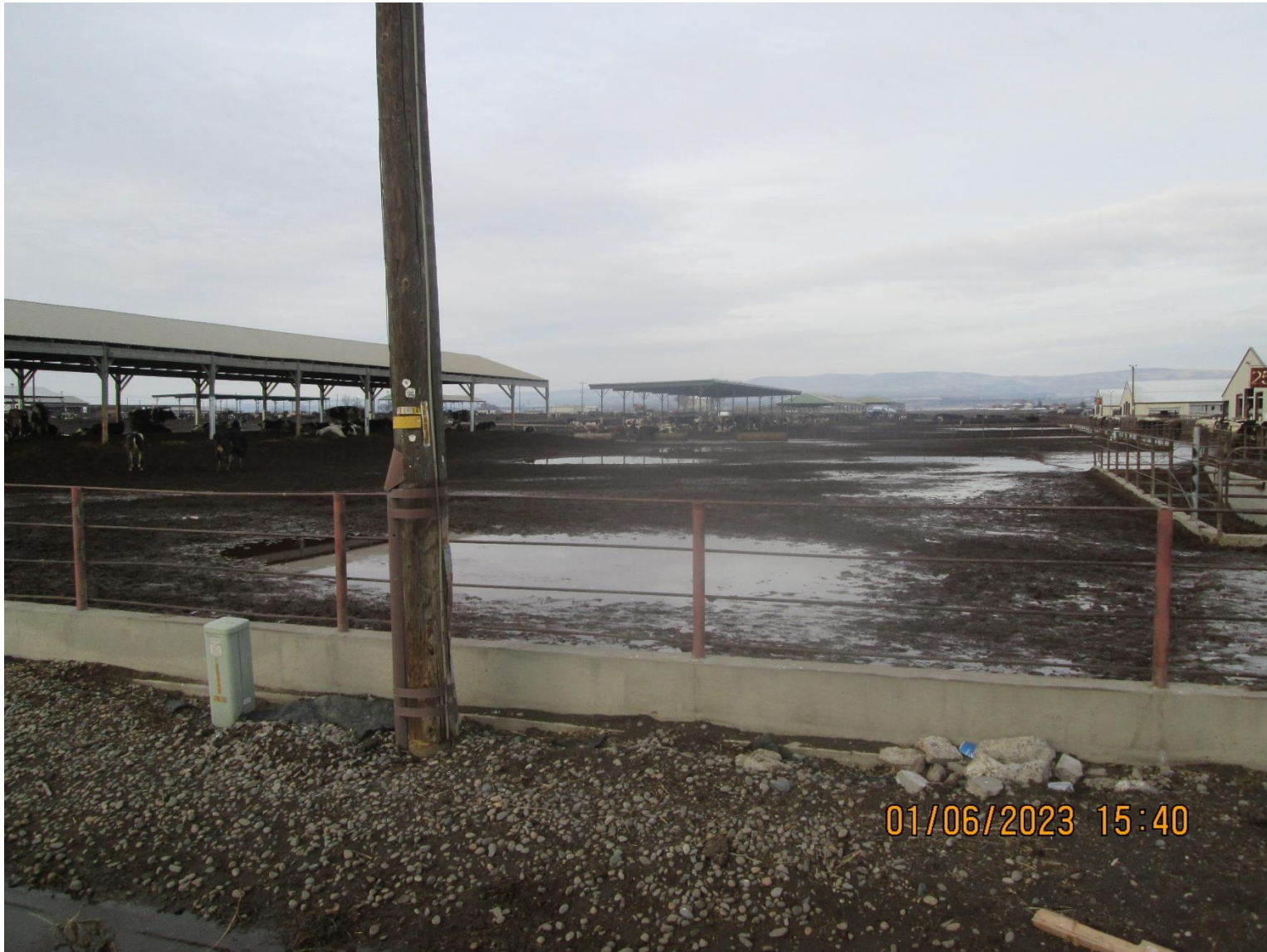
DBD Dairy on Van Belle Road
