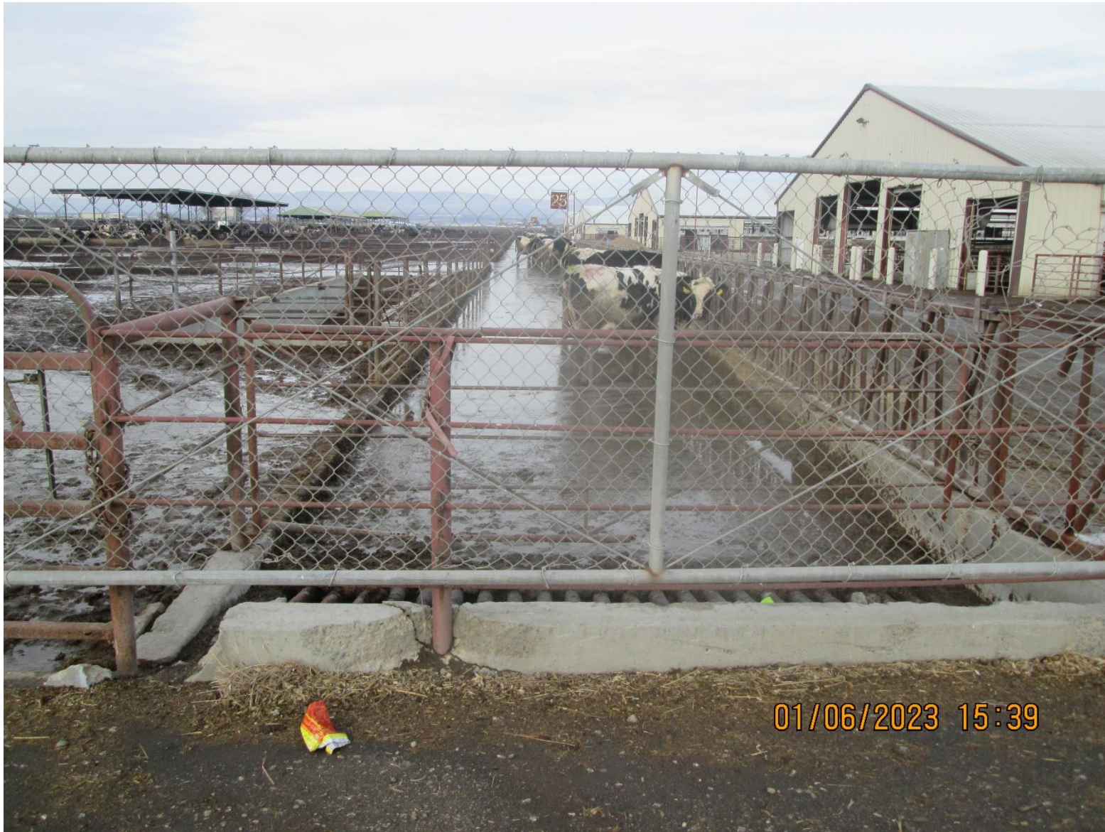
DBD Dairy on Van Belle Road
