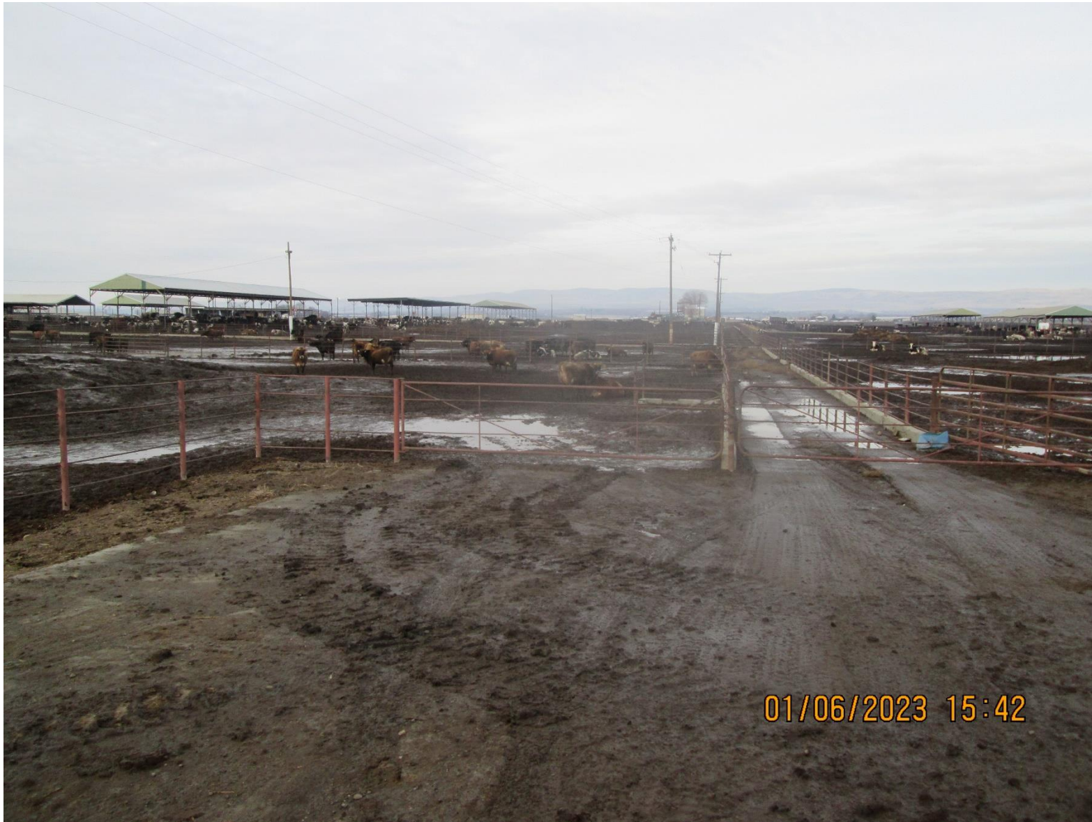
DBD Dairy on Van Belle Road
