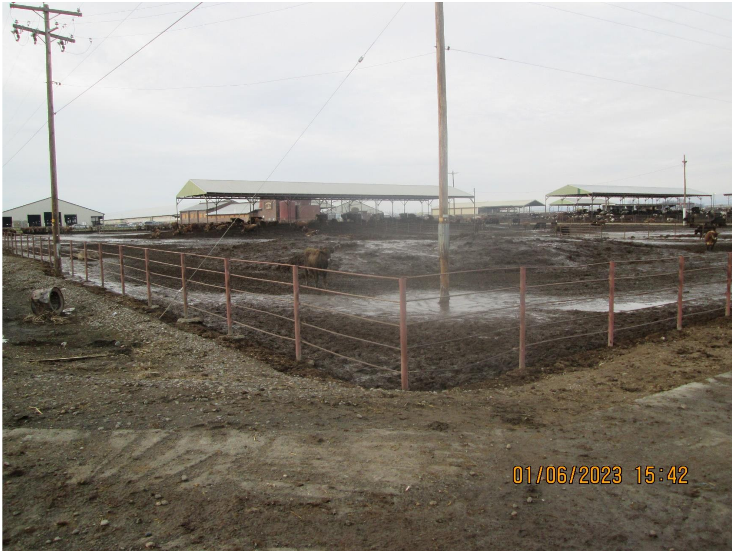
DBD Dairy on Van Belle Road
