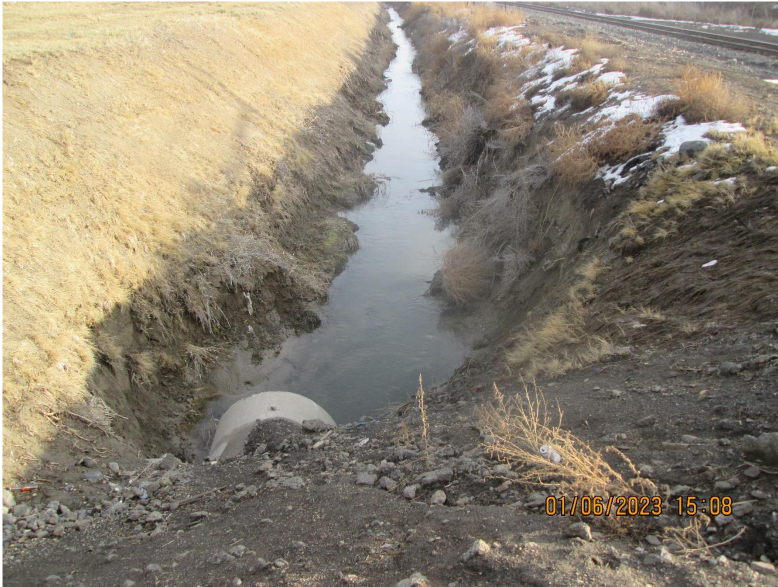
Granger Drain where Gap Road crosses the drain – Looking west
